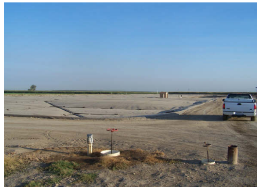
The large primary digester and methane collection pond at Hilarides Dairy in Lindsay
